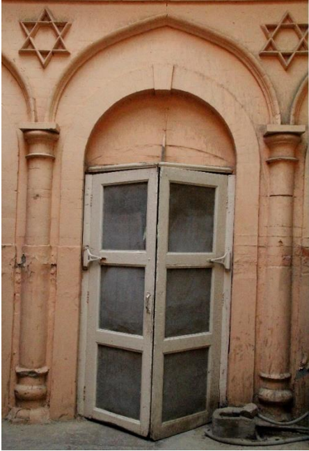
Figure No. 13: Operation Theater.
