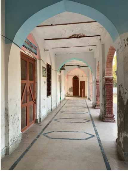
Figure No. 22: Colonnade of SD High School.
