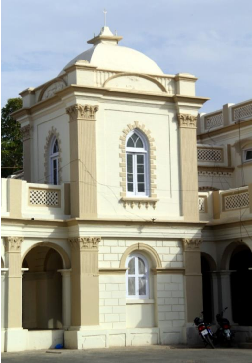
Figure No. 11: Square bastion.
