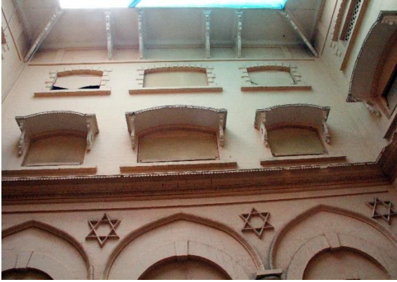
Figure No. 16: Six pointed star and the Chajja of ventilators.
