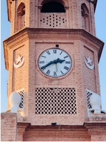
Figure No. 24: Mehrabi motif of central clock tower of SD high school.
