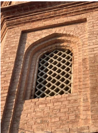
Figure No. 26: Mehrabi motif of the octagonal bastion.
