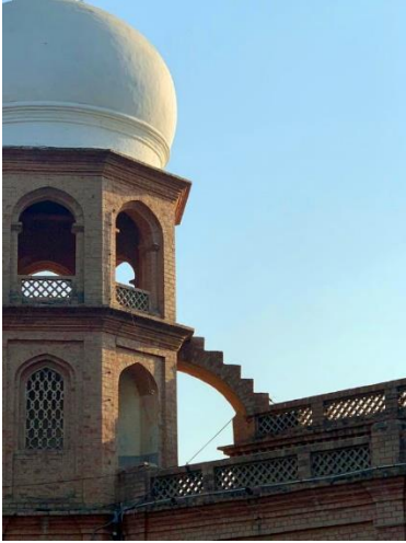
Figure No. 27: Flying buttress of the bastion.
